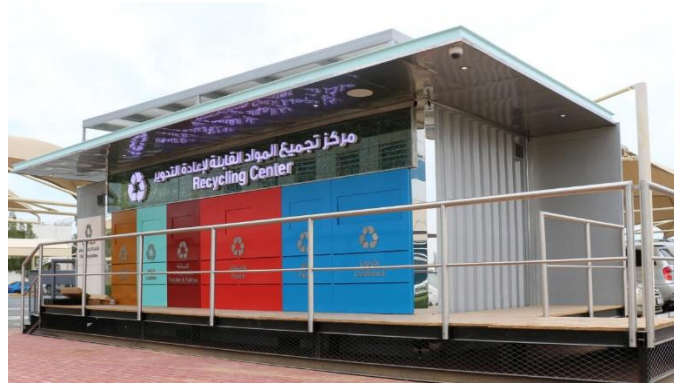
Figure 7: Smart recycling center in Dubai
