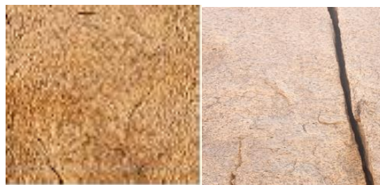
Figure. 1. Ancient Monument Images (a) Normal (b) with Cracks
